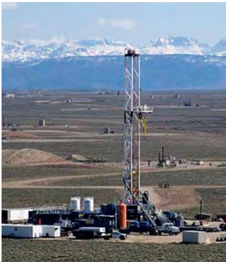
Shale drilling site in Wyoming. Photo: David Mott, U.S. Geological Survey Wyoming Water Science Center, http://pubs.usgs.gov/fs/2012/3049/FS12-3049_508.pdf
